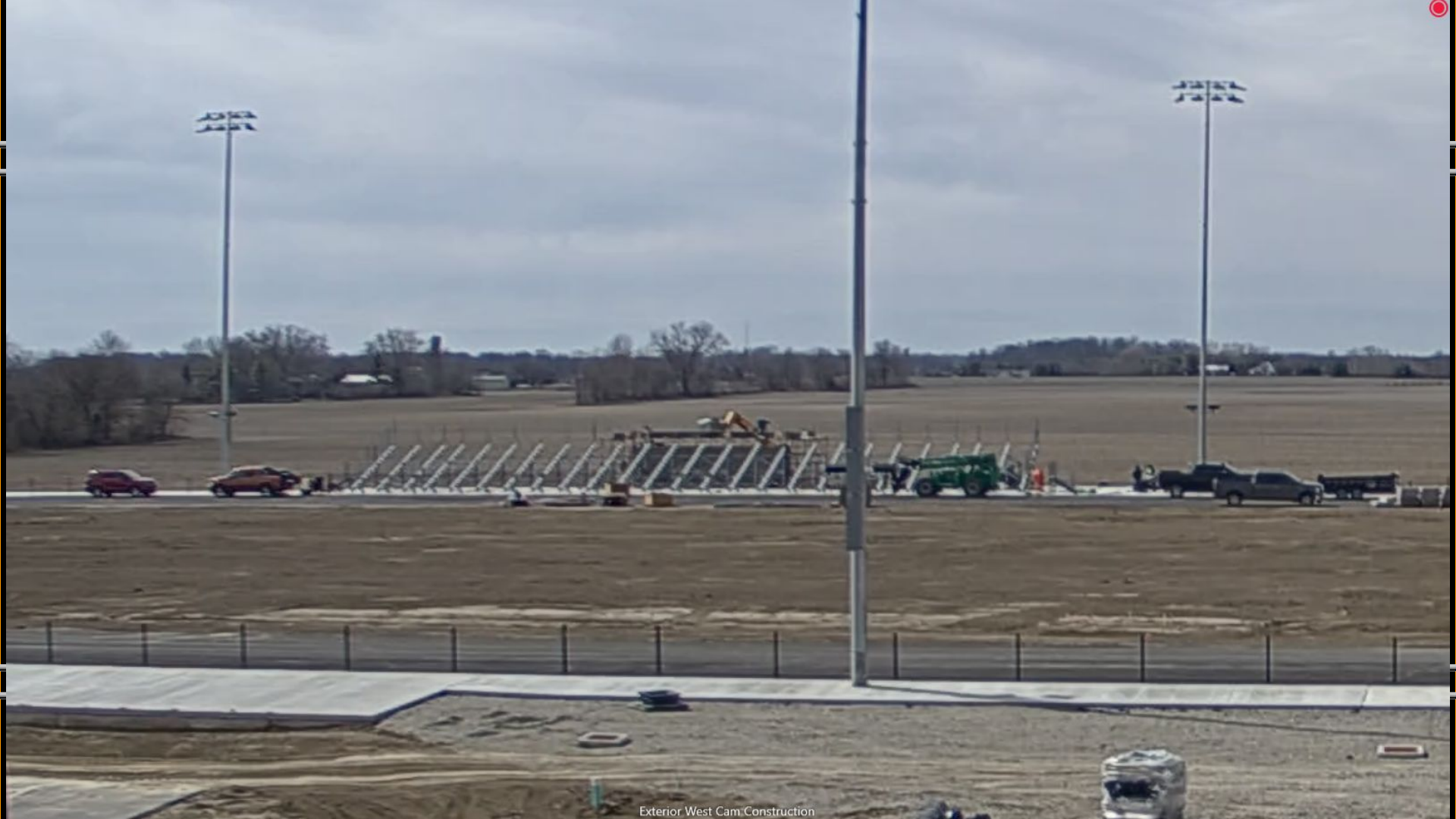
Exterior West Cam Construction
