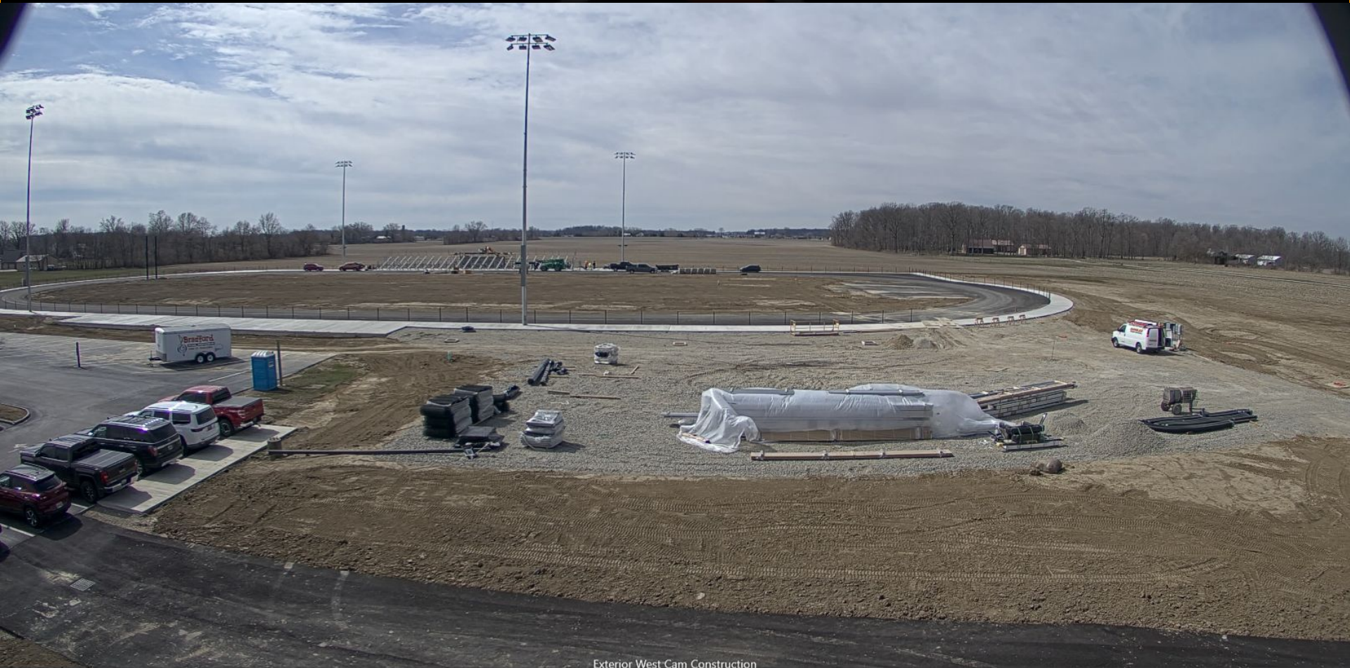
Exterior West Cam Construction
